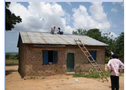
TANZSOLAR INSTALLING A PANEL ON THE ROOF OF A VILLAGE HOME.
